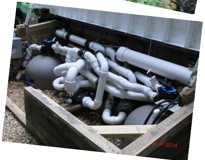
Mike partially buried his filter piping for frost protection
