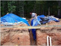
Bill Fricke graciously spent a Sunday afternoon helping to level the site once more. Using a simple water-level (50 foot long 3/8" hose filled with water) we measured and re-measured all around the perimeter. This was a great help in guiding the block layers.
