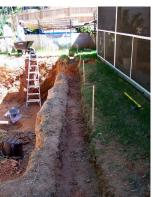
Dual lengths of rebar were laid like a railroad tracks around the perimeter for added strength. Also, at this time we laid a length of 30 amp 4-strand electrical wire in the footer trench, running from the house to the opposite end of the pond where the filter pit would eventually be dug. This wire would be safely encased in concrete once the footer was poured.
