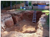
Since we wanted a raised edge for our pond it was now necessary to build a footer for the cinder block wall. We decided on a footer 6 inches deep and 1 foot wide, which meant that first a trench had to be dug all the way around the pond, by hand of course.
