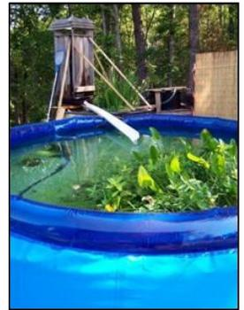
Water is pulled from the main pool using a 700 ghp pump and delivered to the top of the trickle filter. The first 2 drawers have nothing but plastic perforated golf balls. These are the pre-filter sections and need occasional rinsing. Increasingly tighter media is used in the lower drawers which is where most of the biological activity takes place. These lower drawers almost never need cleaning. Filtered water is returned to the tub which then flows back to the main pool.
