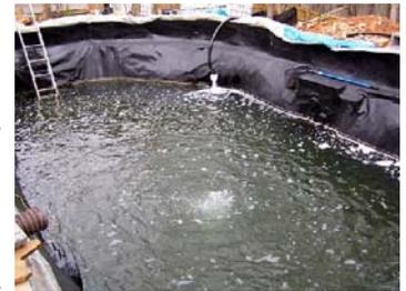
The pond is 1/2 full with all the rains we've had (approx 14000 gal). The flexible black PVC hose you see is output from the sieve. In the middle I'm running one of the air-domes for additional circulation. My plan is to rig the other 2 bottom drains so that I can alternate daily which bottom drain to temporarily hook up to the sieve, and thus clean different areas of the
