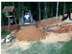
A partial trench was dug near the porch that would eventually connect the main pond to the indoor pond. And a large trench was dug to accommodate the various pipes needed for bottom drains, etc. The completed excavation ended up bit larger than anticipated and came in at 23 feet x 14 feet x 8 feet deep.
