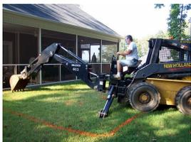
We outlined the area to excavate and Carl started digging. Much rock and hard clay had to be removed. The excavated material was nicely distributed to reclaim some level terrain on sloping sections of our lot.
