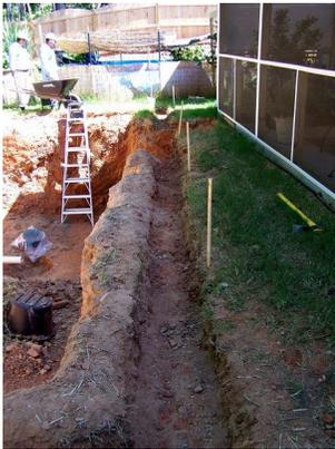
Dual lengths of rebar were laid like a railroad tracks around the perimeter for added strength. Also, at this time we laid a length of 30 amp 4-strand electrical wire in the footer trench, running from the house to the opposite end of the pond where the filter pit would eventually be dug. This wire would be safely encased in concrete once the footer was poured.
