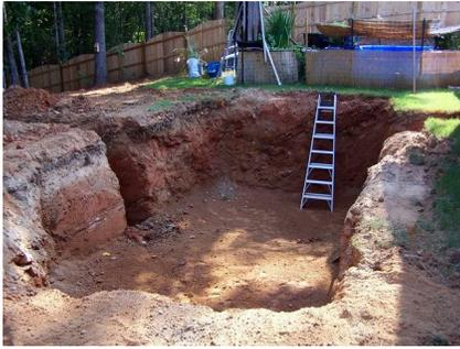
Since we wanted a raised edge for our pond it was now necessary to build a footer for the cinder block wall. We decided on a footer 6 inches deep and 1 foot wide, which meant that first a trench had to be dug all the way around the pond, by hand of course.
