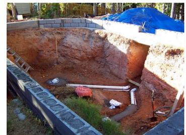
The finished dimensions of the pond, measured from the inside wall edges ended up being 27 feet long x 16.5 feet wide x 9 feet deep (yep, forgot to add the height of the wall before). That equates to more than 29,000 gallons in a perfect rectangle! Since we designed one side to be at a diagonal to accommodate a waterfall, both this and the sloped walls would reduce the eventual volume of the pond.
